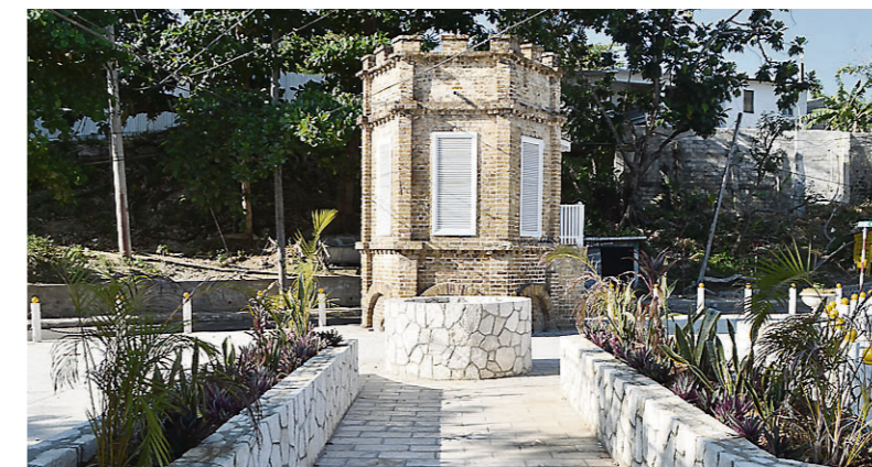
The Montego Bay Dome, which was rehabilitated by the Tourism Enhancement Fund.
